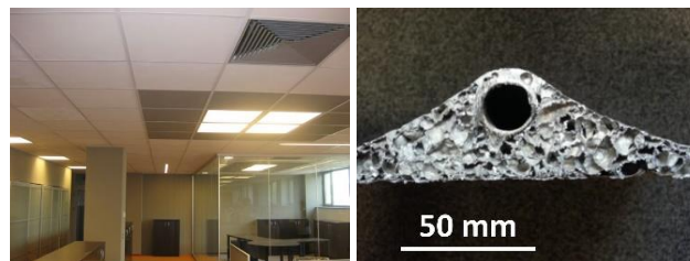
Fig. 4. Ceiling aluminium foam radiators in the open office space area 260 m 2 of company Hydro Extrusion Slovakia JSC in Žiar nad Hronom, Slovakia (right – cross-section of aluminium foam structure with embedded tube distributing heat transfer fluid).
