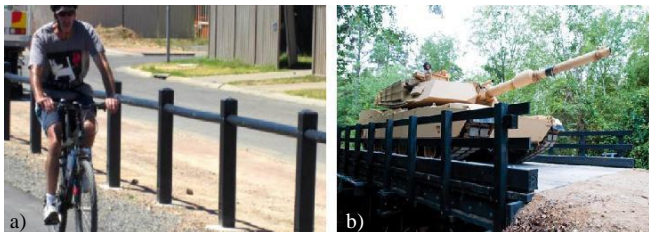
Fig. 1. a) Fencing made of recycled plastic in South Australia (1); b) completed T-8518 bridge made of recycled plastic at Fort Bragg, NC (Source: U.S. Army) ; c) cut of a standard recycled plastic beam [16].
