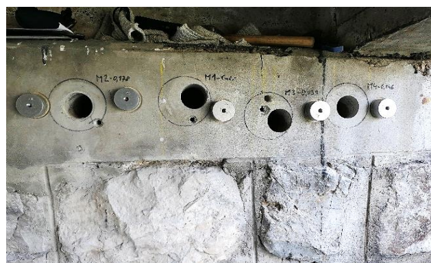
Fig. 2. Device for the on-site measurement of surface tensile strength.
