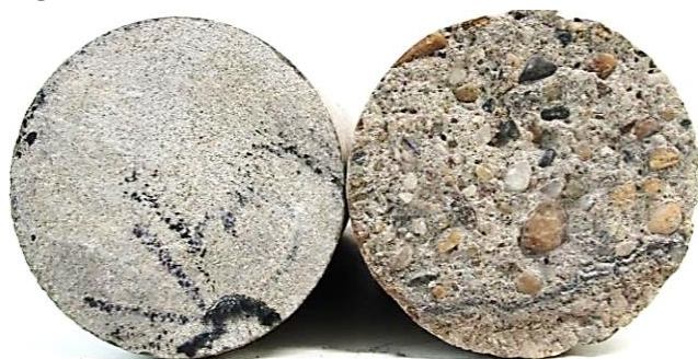
Fig. 6. Concrete from the bridge Sládkovičovo covered (left) and uncovered (right) by the PRC.
